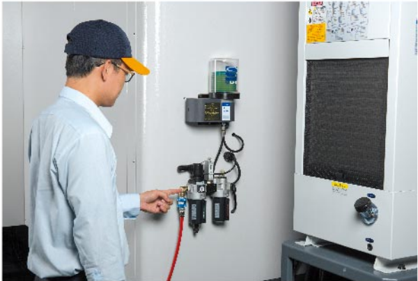
Through centralized management of air FRL unit and lubricant pump, daily maintenance is made easily.
